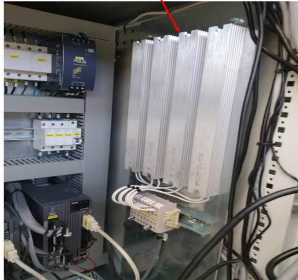
Figure 9: Resistor for Energy Recovery of the External Axis.
