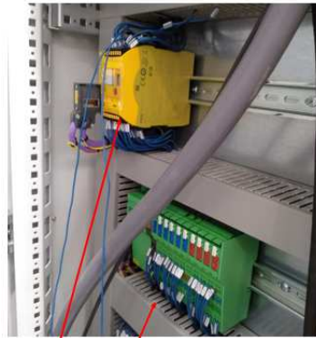
PLC—PILZ OF DIGITAL INPUT (BLUE CARD) AND OUTPUT BOT
